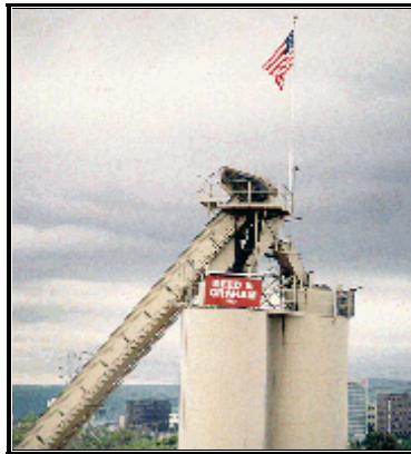
Asphalt storage bunkers, San Jose facility
